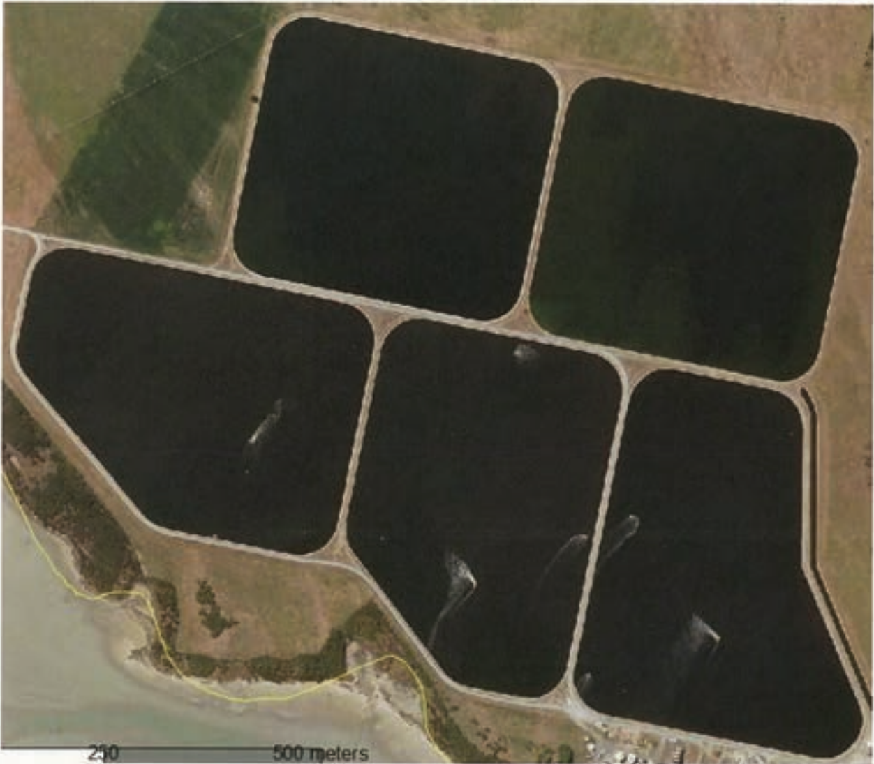
Bell Island WWTP Aerial View
